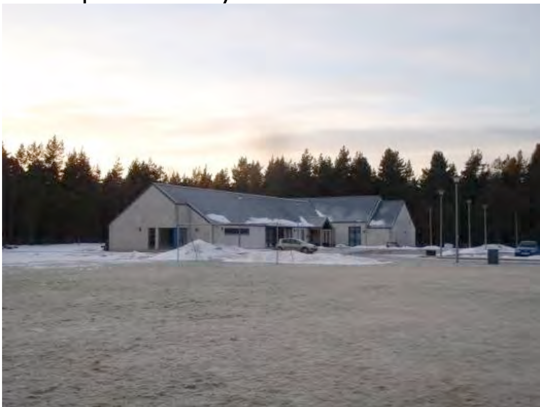
Figure. 4- Boat Community Hall site behind hall
